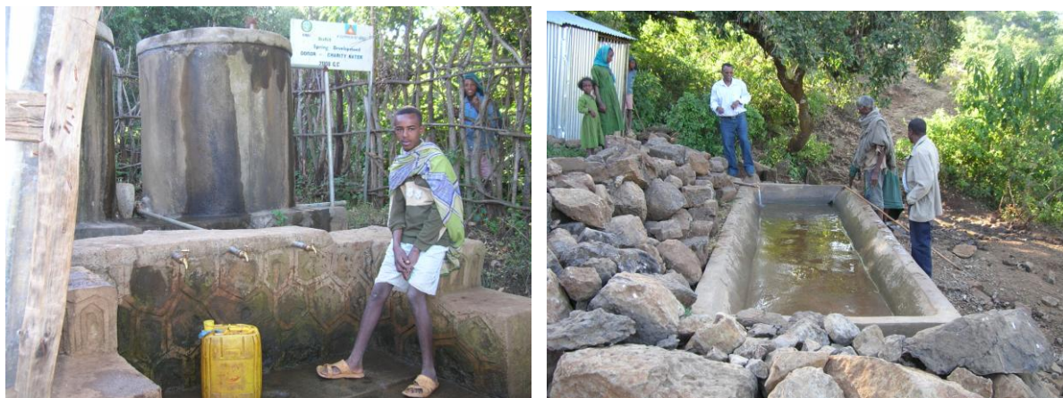
Figure 2.3. Water Infrastructures in ANRS [pictures taken by Mina Noor]
